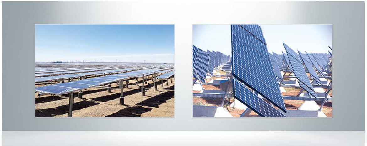
Figure 1. PV Uniaxial Tracking Device PV Double-axial Tracking Device
